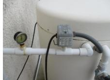
5) **Slowly** pull the 'L' shaped lever switch up until you hear water or a pump start to run and then hold it in that position. As you are holding the switch, listening to the water/pump run watch the pressure gauge needle start to rise. When the gauge needle reads between 40-45 let go of the switch. The water/pump should continue to rise by itself at this point and will shut off automatically.
